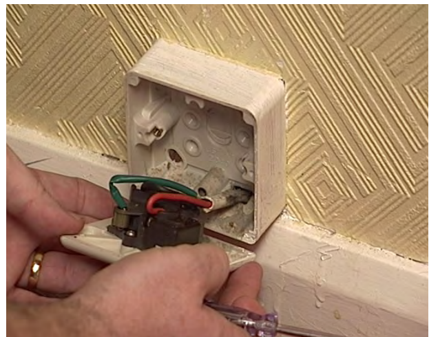
Inspecting a socket-outlet
